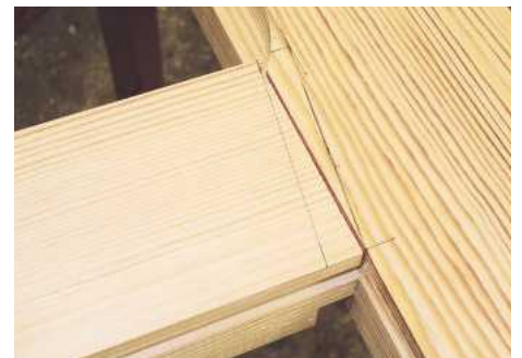
▲ Pic.7 The diminished shoulder on the outside centre rail...
